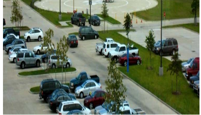
Houston, Texas Park and Ride parking lot. I-10 Katy Freeway park and ride lot in Houston, Texas. Photo courtesy Shishir Shishodia.
